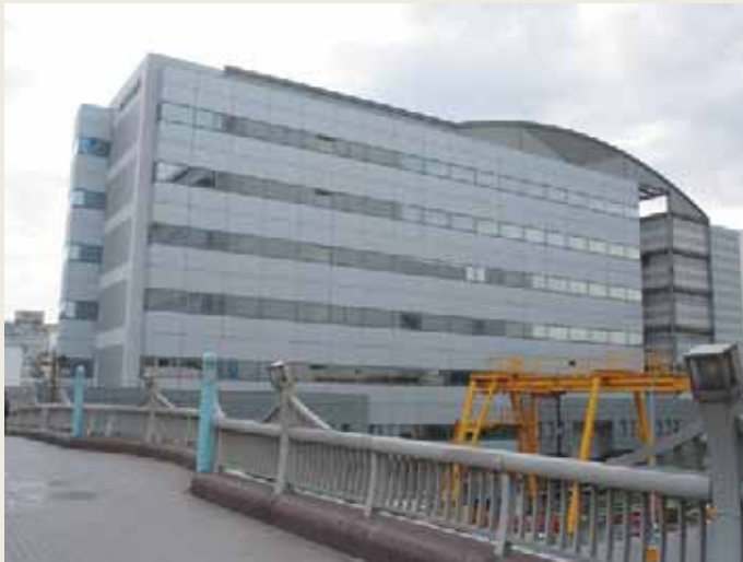
The Chiba Tech Building, east of Tokyo and accessible to Narita Airport, is Rotex's base of operations in Japan.
